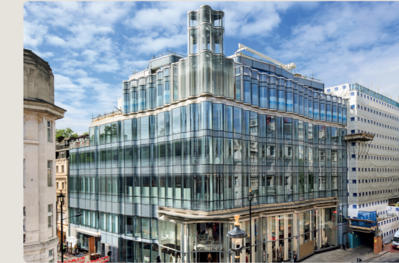
4 61 Oxford Street W1 35,000 sq ft retail space, 14,000 sq ft office space, 6 residential units
